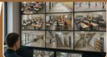
24x7 CCTV Surveillance & Warden Supervision
